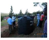
The water pipe passes through farm land adjacent to the school site. The pump can fill the 5,000 litre header tank in one hour. The water will be gravity fed to a stand pipe near the kitchen and into the girls washroom, where it will feed a shower. Eventually it will also provide piped water to the science lab.
